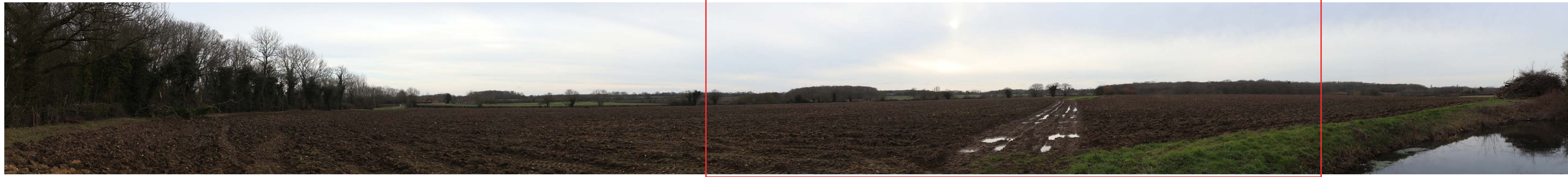
Site Context Photograph (2 of 2)
